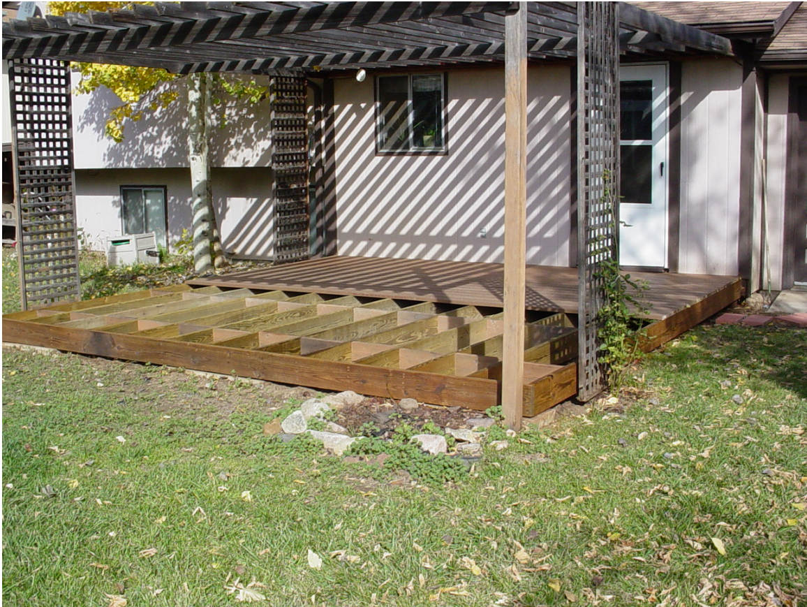
New 2X8 pressure treated stringers set on pavers
