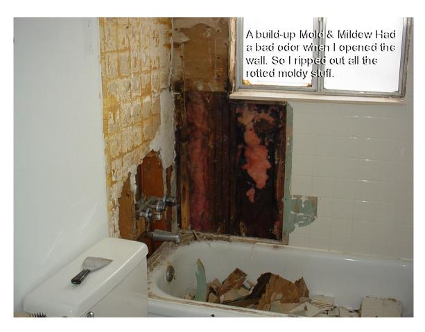
The studs in the wall around the window were rotted and the wall would need to be rebuilt.
