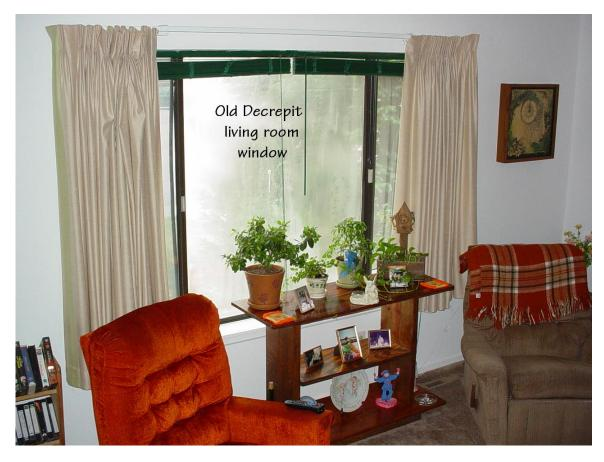
The seal had deteriorated letting moisture in between the glass
