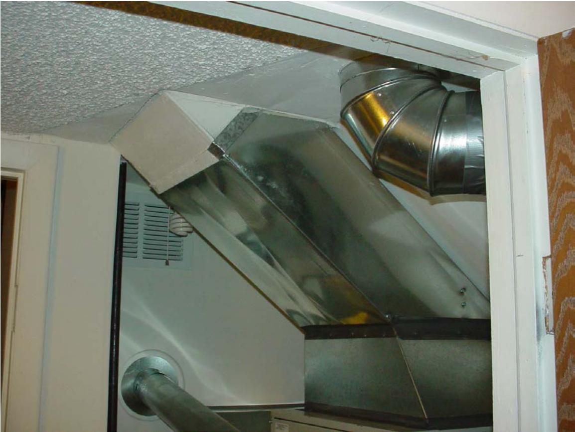
Also incorporated an electrostatic air cleaner in the return
