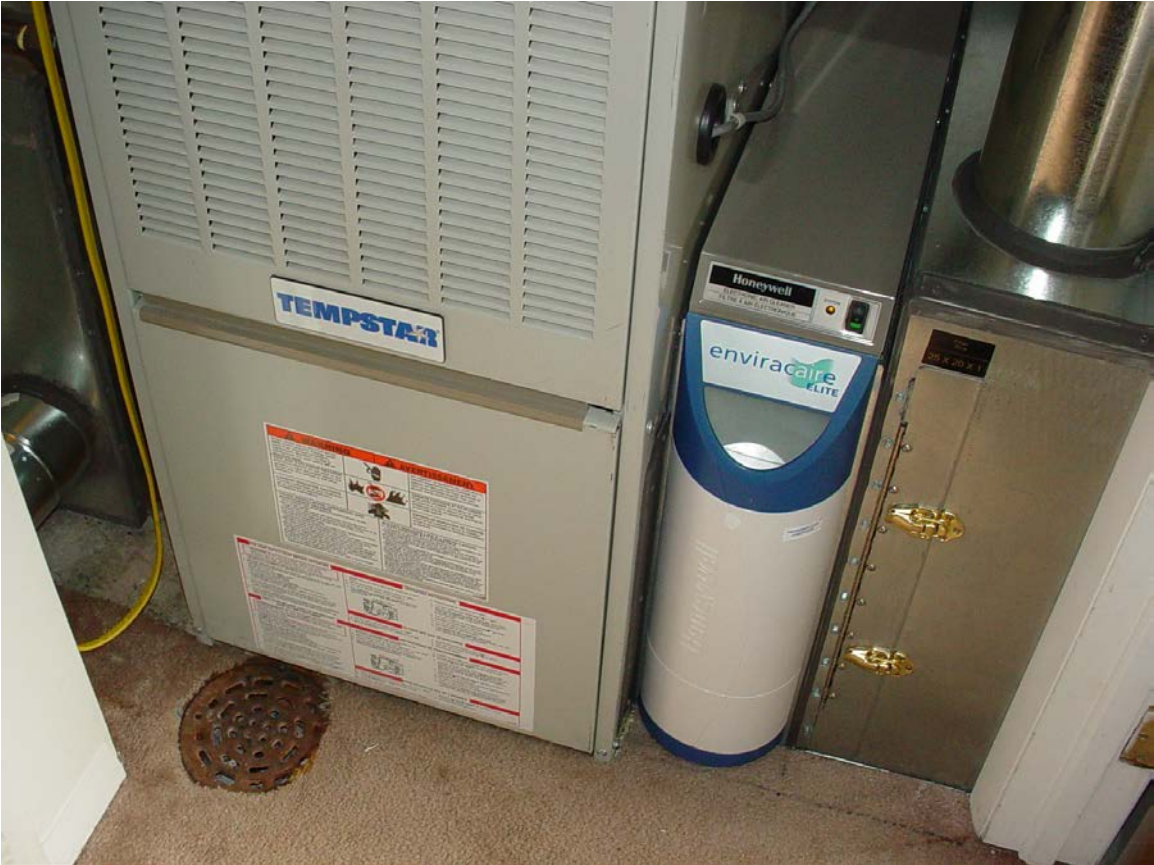
Also incorporated an electrostatic air cleaner in the return
