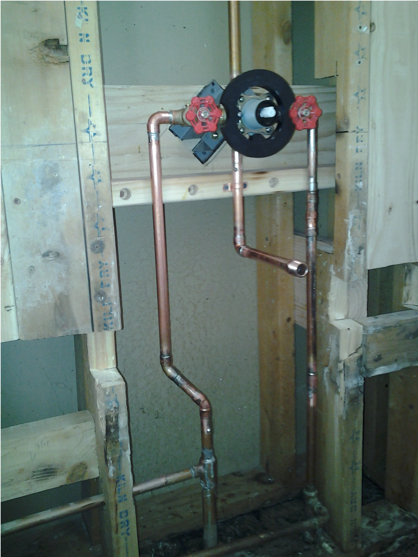
Time for the new plumbing
